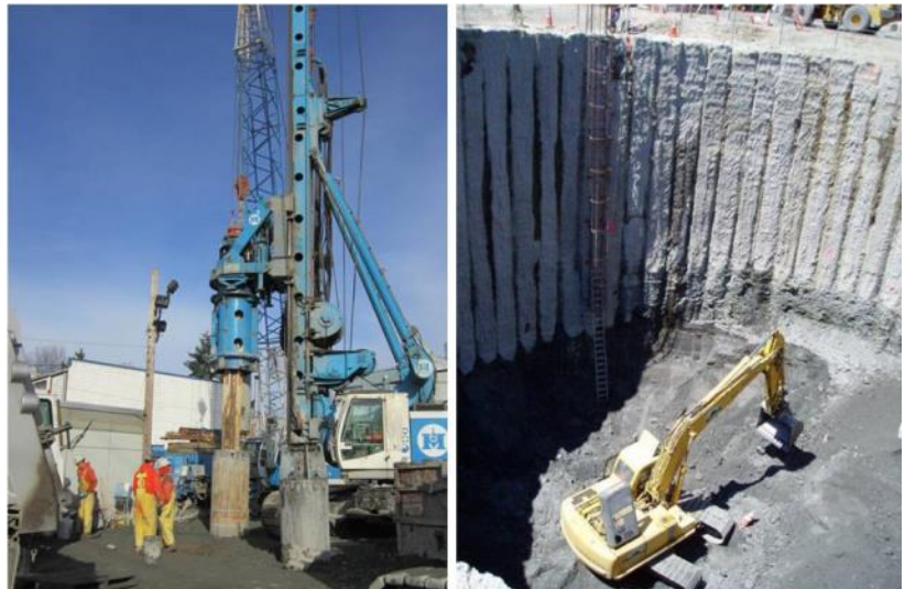
Secant piles interlock to create a watertight ring that controls groundwater.
