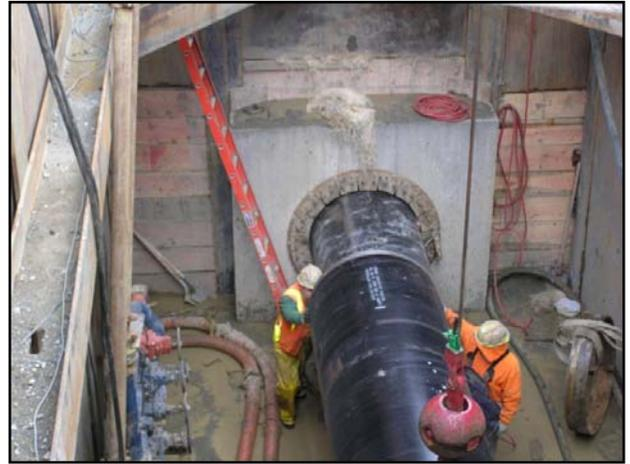
*Pipe sections are fed through the launch shaft*
