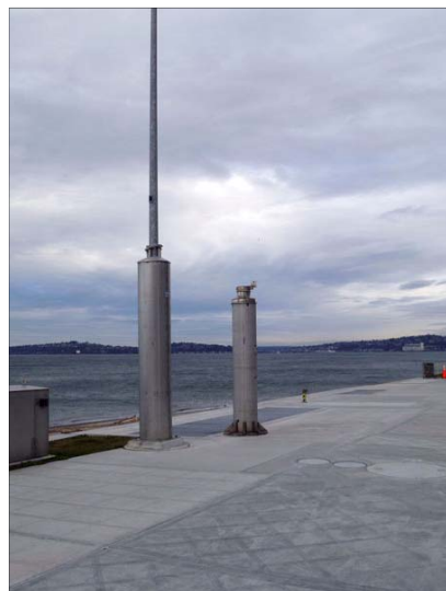
53rd Avenue Pump Station, Alki Beach, West Seattle
