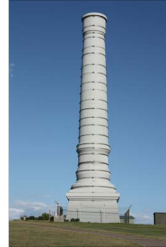
North Bondi sewer vent, Sydney, Australia
