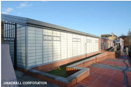
Translucent fiberglass panels
