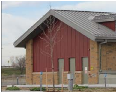
Metal and CMU siding
