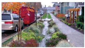
After a big rain, wetlands and bioswales clean the water and allow it to soak into the ground over several hours.
