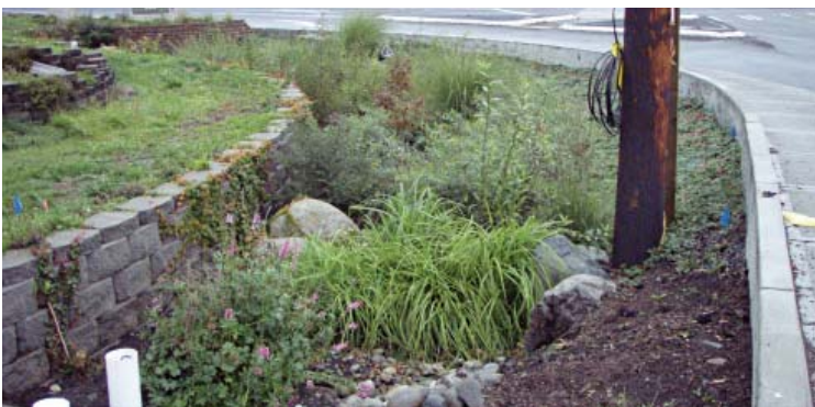
A low impact rain garden at the intersection of South 272 nd Street and Military Road South. This low impact strategy uses a planted depression that allows stormwater to soak into the ground rather than to run off into the storm drain.
