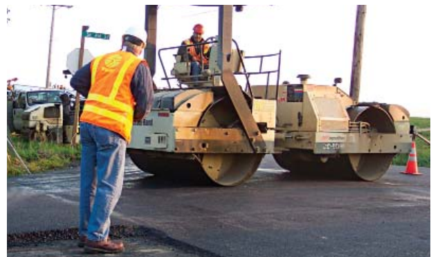
A Washington State Department of Transportation employee inspects the experimental RAS paving.
