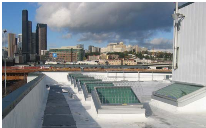
Ryerson Base skylights for interior daylighting.
