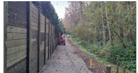
Constructed in 2011, a sound barrier wall along the west side of the transfer station helps reduce noise impact to neighbors
