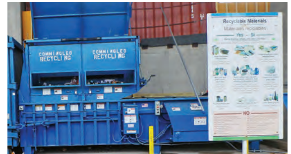
Compactors for recyclable materials
