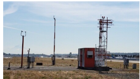
The Runway 14R glideslope antenna and tower, which is expected to be replaced by the FAA this month
