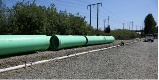
A crew member inspects a dewatering pipe. This pipe removed groundwater during construction to allow crews to successfully install the green force main pipe underground.
