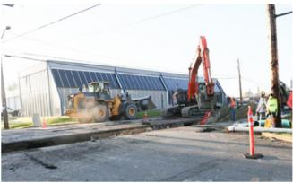
Crews dug a trench to install pipe underneath Frontage Road in Pacific.
