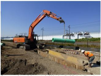
Crews used trench boxes to hold back soil while installing pipe alongside Perimeter Road in Auburn.
