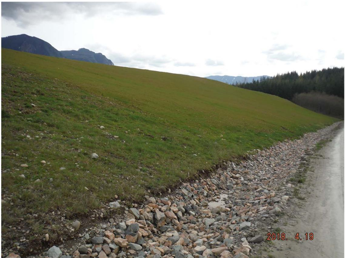
**Photo 3A.** Rock-lined ditches are constructed at the base of backfill slopes to convey storm water to one of three infiltration ponds.
