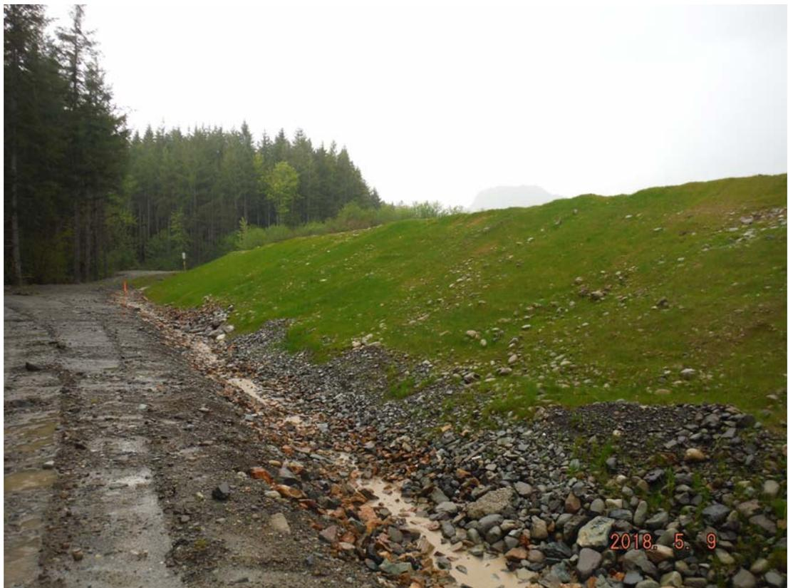
**Photo 3B.** Newly constructed perimeter berm and drainage ditch along revised permit boundary. Here the ditch defines the permit boundary with the forest access road along its outside edge.
