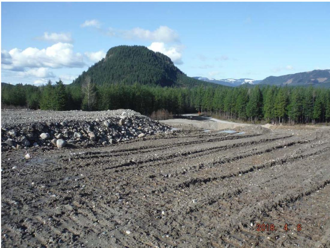
**Photo 2A.** Once the backfill soil has been pushed into place, a driving surface consisting of a 2-3 foot thickness of pit-run gravel is placed to allow dump truck access to allow further soil dumping to advance the fill prism.
