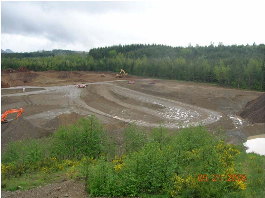
**Photo 1A.** New mine segments are stripped and grubbed followed by mining pit-run gravel to 40-feet below the existing grade.
