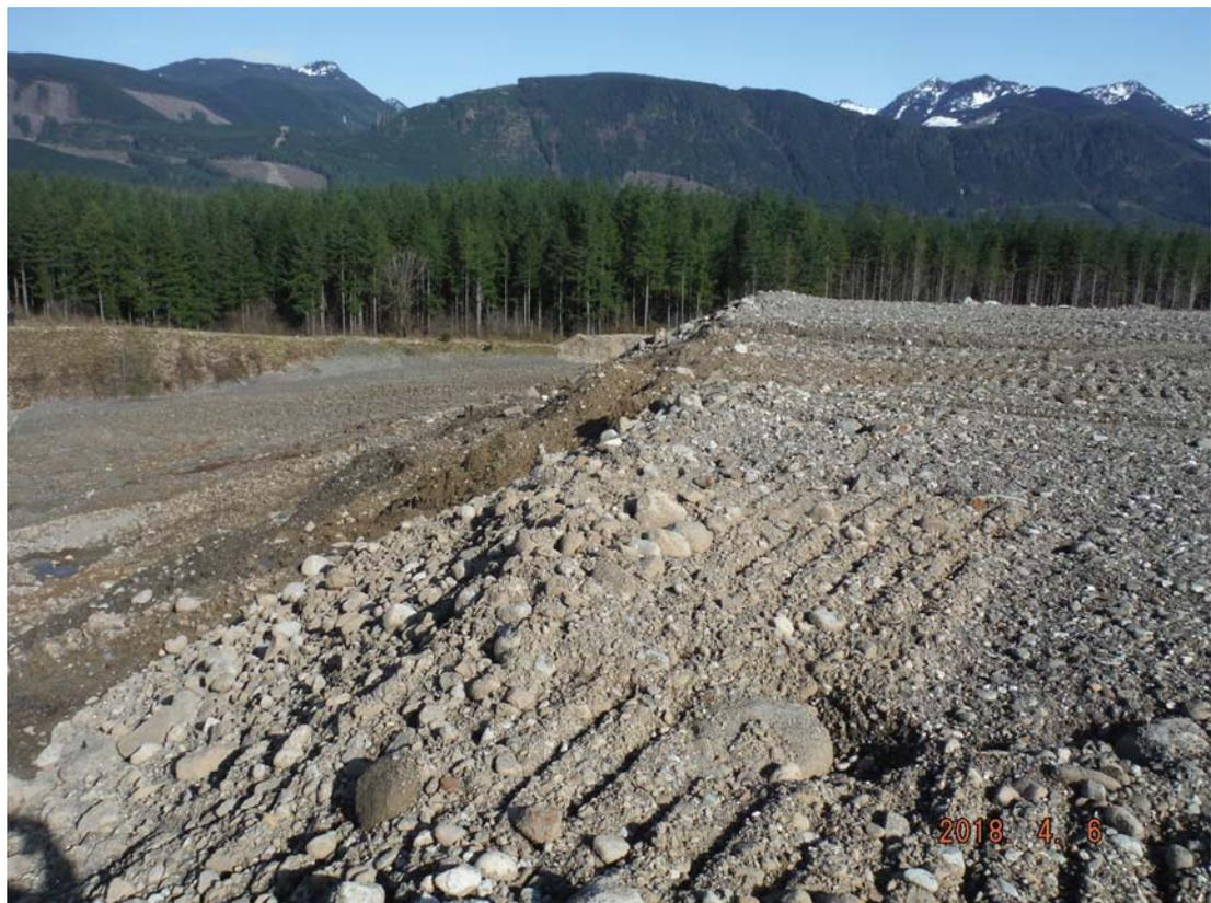
**Photo 1B.** Following pit-run mining, backfill soil unloaded by dump trucks and placed by bulldozer into the mined out segment. Up to a 80-foot thickness is placed to backfill the pit and raise the final floor elevation to 40-feet above pre-existing grade.
