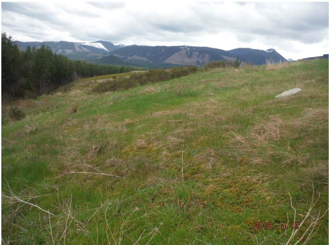
**Photo 2B** Final backfilled slopes are seeded with deep rooted grasses and forbs to stabilize soil and limit erosion. Eventually the site will be planted with trees and revert to commercial timberland.
