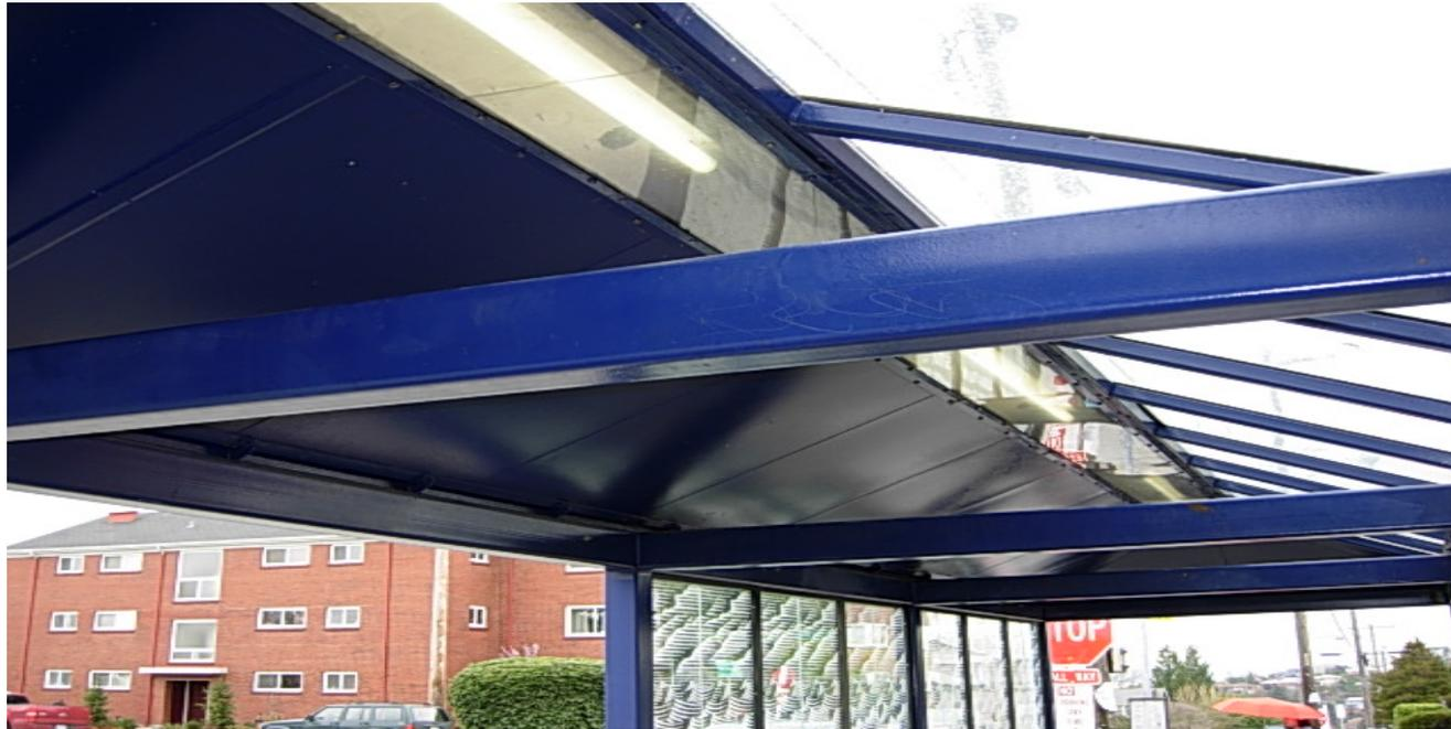
In the late 1970's, Power and Facilities began installing fluorescent lighting in bus shelters throughout King County. At the time, it was the most economical and reliable method of lighting bus shelters available. After a number of years, re-lamping and repairing these light fixtures became expensive and time consuming. Something better was needed...
