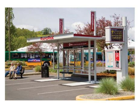
**RapidRide:** RapidRide shelters are prefabricated from durable steel frames that will be refurbished every eight years, with an estimated life of 35 to 40 years. Replacement shelters get reused for other routes.
