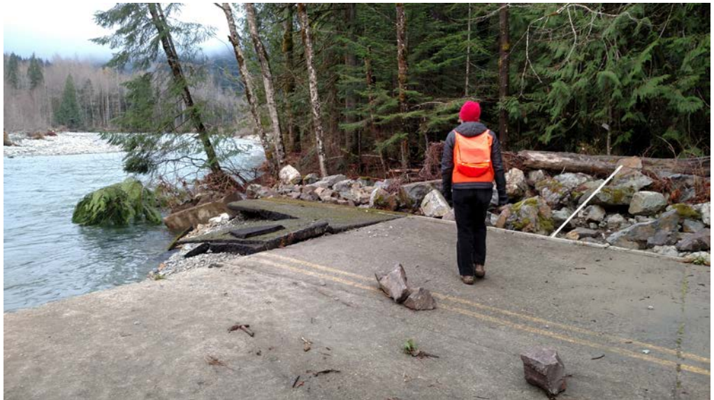
Exhibit G: Flood monitor inspecting damaged road near town of Skykomish.
