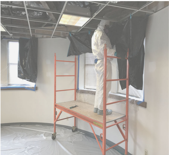
Exposure monitoring during lead abatement work by utilities workers
