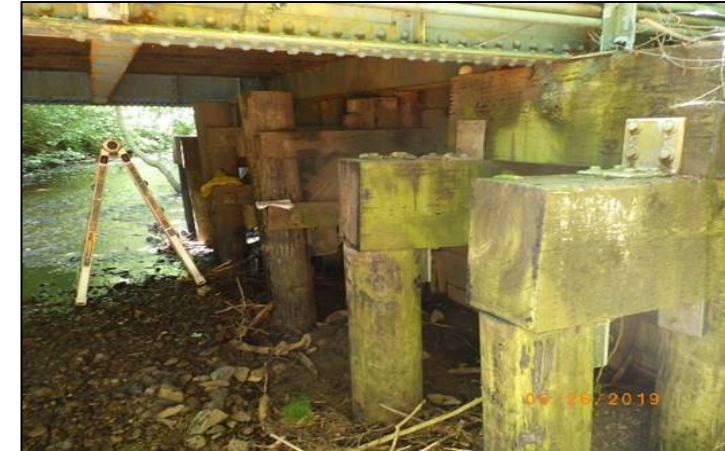
Coal Creek Bridge girders (left) and abutments (right)
