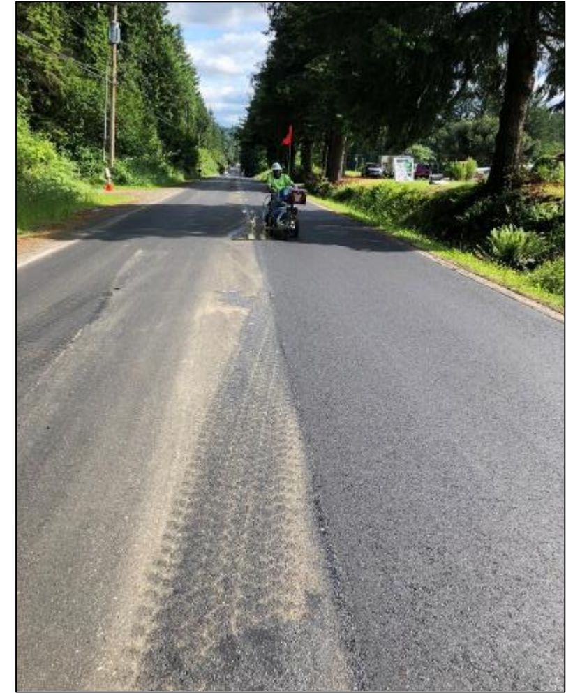
BEFORE and AFTER: Pavement preservation at 244th Avenue SE from SE 200th Street to SE 192nd Street.
