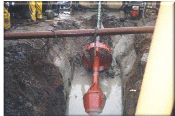
Specific equipment is used for drilling in different conditions. Both drill bits and reaming heads for the Magnolia Project will be selected based on the soil types found at the drill depth
