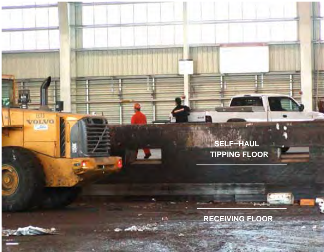
Figure 11 – Typical Grade-Separated Self-Haul Tipping Floor Above Waste Receiving Floor
