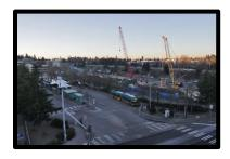
**Parcel** # **292604-9025-** Construction of the new 236,684 sf Northgate Mall Parking Garage located at the west side of the mall at 301 NE Northgate Way is well underway. The new structure is a two-story parking garage with 673 stalls and an adjacent surface parking lot with 137 spaces will be re-striped.
