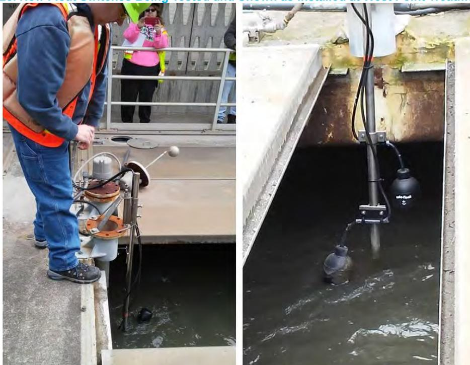
Because these float switches are not intrinsically safe (electrical spark/ignition limiting) and the area in which the float switches are located has been identified as hazardous, an intrinsically safe relay was also added for each float contact before interfacing with the Ovation control system or the RSP interlock circuit. These new float switches have been successfully tested at WPTP and the County has now adopted them as its new standard for float-level switches at all plants.
