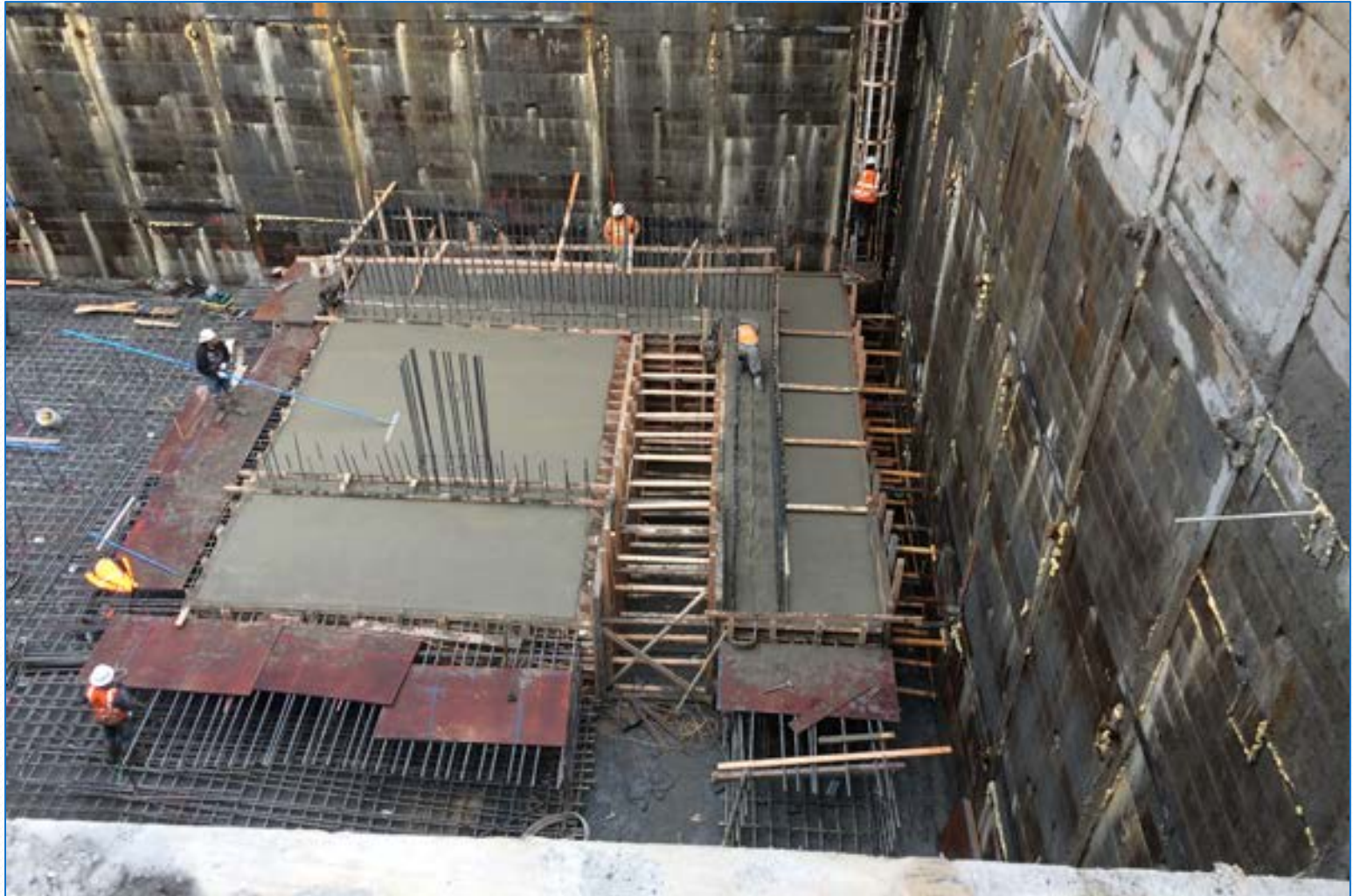
Base slab for Rainier Valley storage tank
