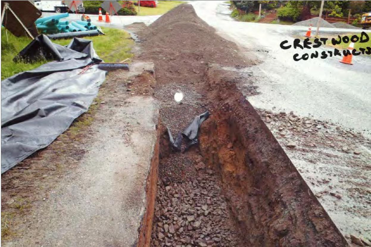
Figure 2-3. Retrofit Trench Drain Captures Groundwater Flow and Alleviates Pavement Settlement
