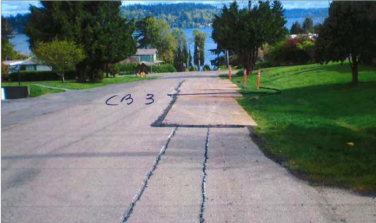
Figure 2-1. Pavement Settlement Along Sewer Main Alignment Following Construction
