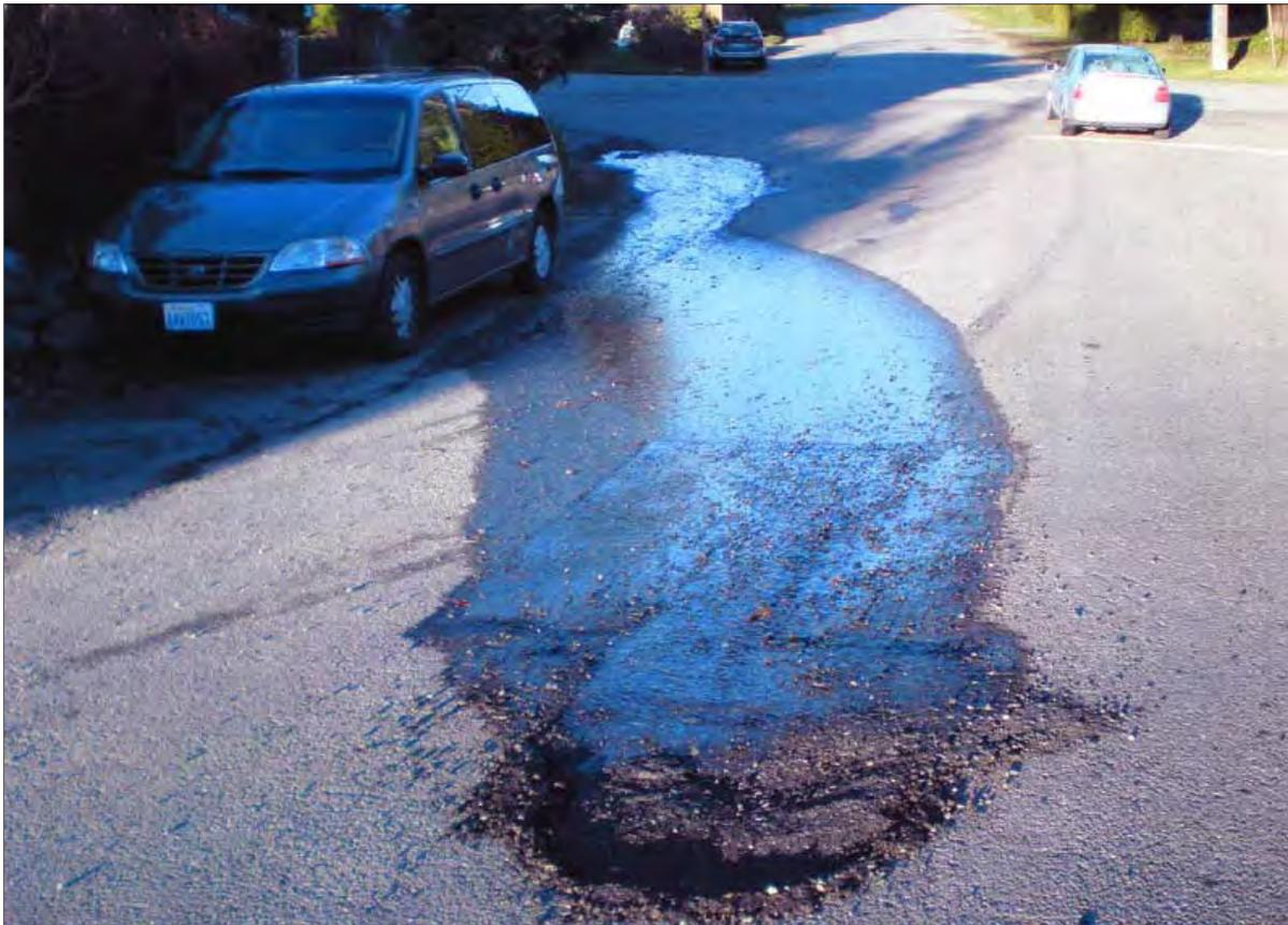
Figure 2-2. Groundwater Following Burst Sewer Main Trench Breaks Out of Pavement
