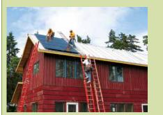
Solar PV system being installed on a metal roof. Source: Studio Hamlet Architects.
