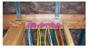
In an addition, new construction or a gut remodel, there are many opportunities to seal electrical penetrations and top and bottom plates. Source: O'Brien & Company
