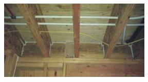
Air sealing with expanding foam or caulk at a rim joist is an effective means of sealing leaks. Source: O'Brien & Company
