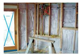
This picture shows the "flash" portion of a "flash and batt" installation. The flash coat of spray-in-place foam insulation creates a tight air seal. Source: O'Brien & Company
