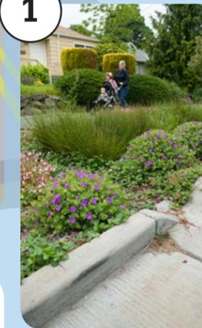
Roadside rain gardens absorb large amounts of stormwater from streets and sidewalks. They are typically located in planter strips and work best with a moderately sloped street – they need water to flow downhill so that it can be easily diverted into the garden.
