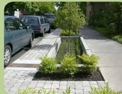
Tree boxes are street trees designed to store and filter stormwater. They work well in small spaces and provide multiple benefits including reducing air pollution and absorbing carbon dioxide.
