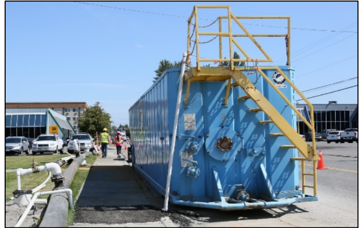
Dewatering tanks and pipes will be reinstalled.
