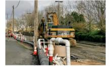
**Dewatering:** installing a series of wells and pipes along the pipeline route so that groundwater can be temporarily removed. This allows the soils to be stable enough to install the pipeline.
