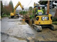
(trenched) pipeline construction: a section of pipe is placed in a trench, then covered, before moving on to the next pipe section.
