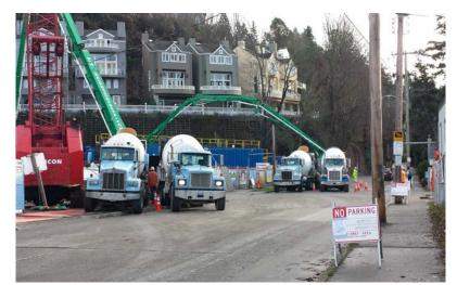
Two pump trucks will pump concrete into the hole from Beach Drive S.W. on pour days.
