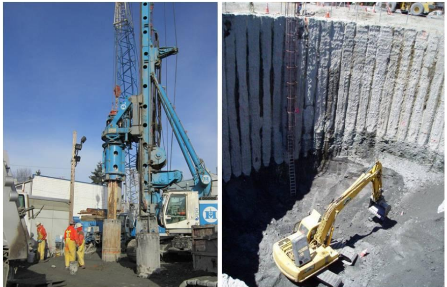
Interlocking secant piles create a watertight ring that will form the outer wall of the storage tank.
