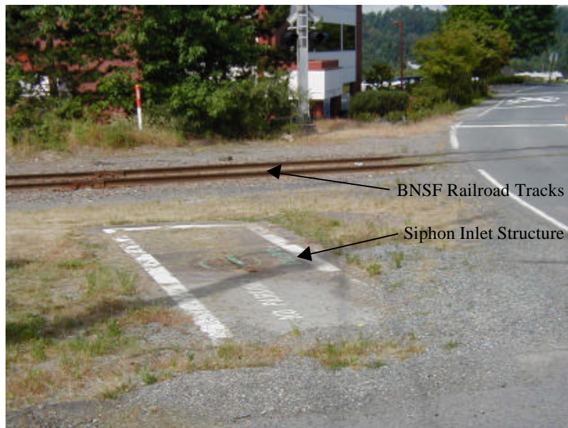
Figure 2-4: Existing Wilburton Siphon Inlet Structure
