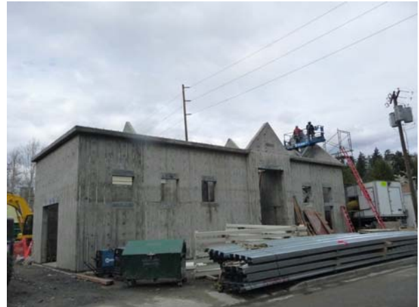
Steel decking for new roof of Bellevue Pump Station, March 2010
