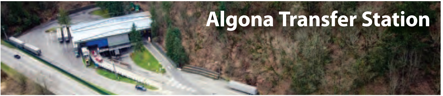
Aerial view of Algona Transfer Station
