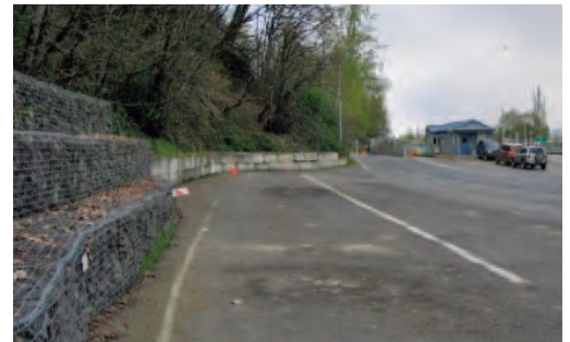
A gabion wall helps prevent damage from mudslides.
