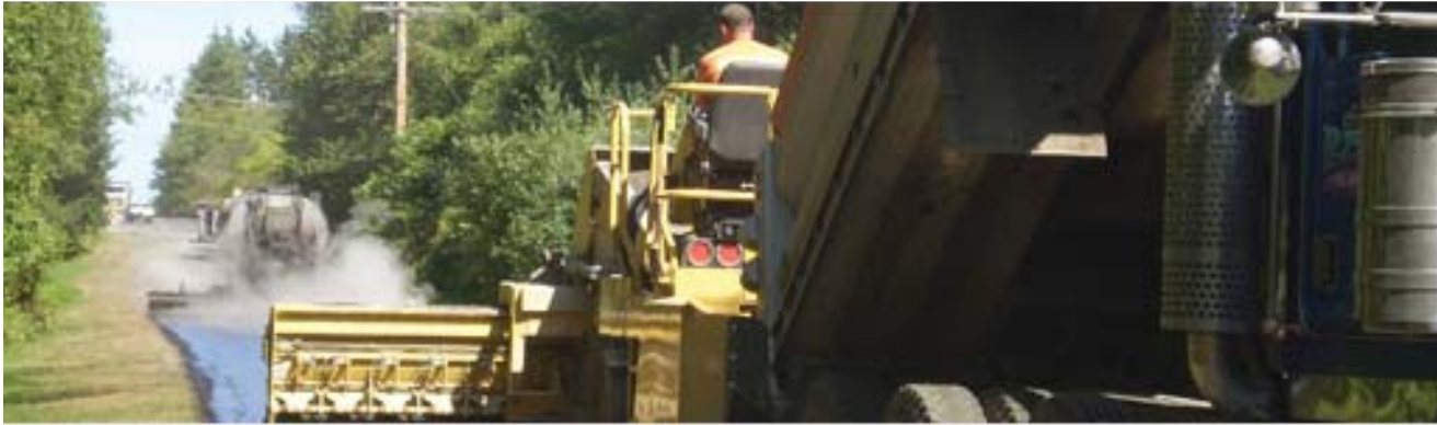
Chip sealing a rural county road
