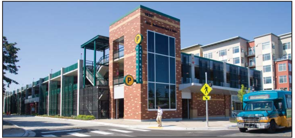
The new Redmond Park-and-Ride Garage, above, was designed to fit in with the multi-use building next door (visible on right).
