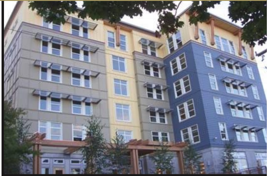
Building Green - Evans House in Seattle provides 75 studio units of permanent supportive housing for chronically homeless and mentally ill adults, including 4 units set-aside for persons with developmental disabilities. It was built using energy efficiency and sustainability standards, as well as universal design elements for accessibility.
