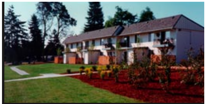
Laurelwood Garden in Federal Way - Renovated by the King County Housing Authority to provide 92 households with affordable housing, a safe place for children to play, and a sense of community.
