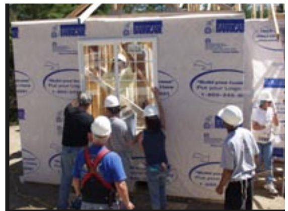
Ron Sims (placing window) working with Habitat for Humanity in Snoqualmie
