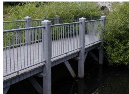
Meadowbrook Pond Bridge
