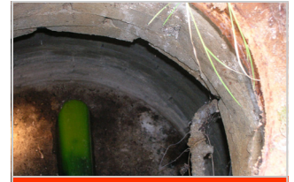
Green dye in sewer from burrow
