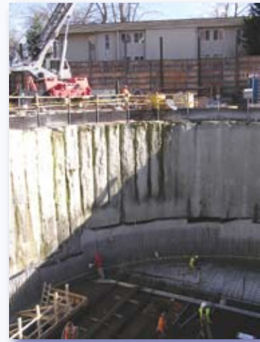
New pump station under construction
