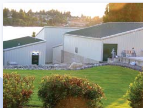
CSO treatment facility in Bremerton, WA, showing top of underground storage tank on the right and treatment building
