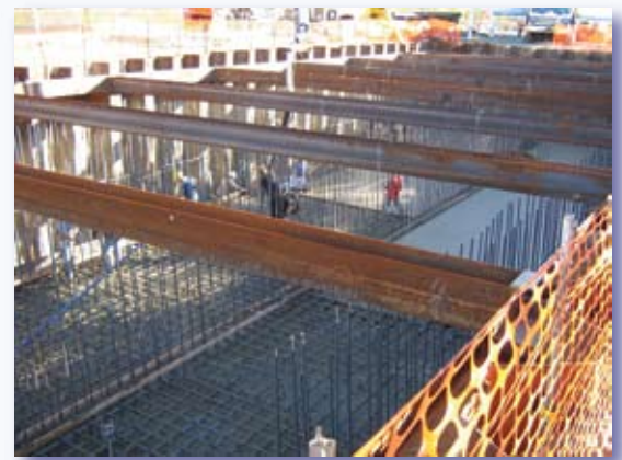
Excavation nearly complete for a 400,000 gallon storage tank in Blaine, WA
