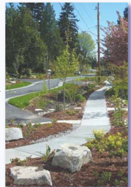
A bioswale stores and filters storm water runoff
