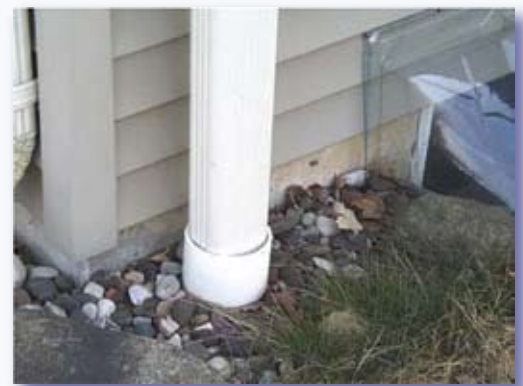
Downspouts are directly connected to combined sewers in older cities like Seattle
