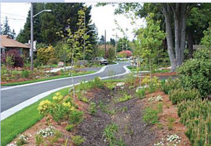
A bioswale stores and filters storm water runoff
