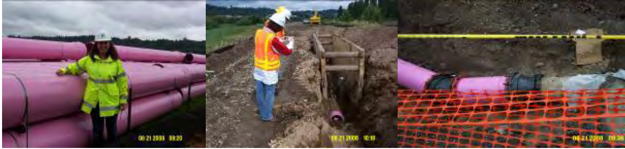
Figure 9. Construction of Brightwater South Transmission Line
