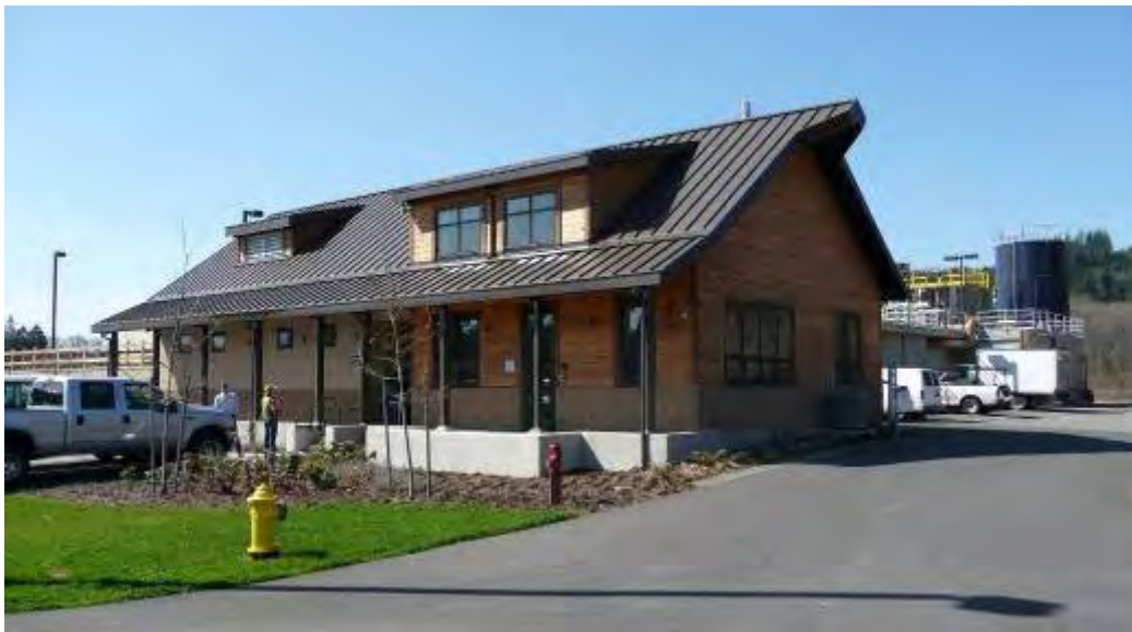
Figure 6. Carnation Treatment Plant
