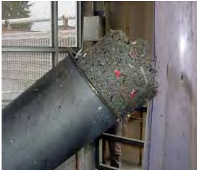
South Plant screenings material that has been processed with a washer compactor
