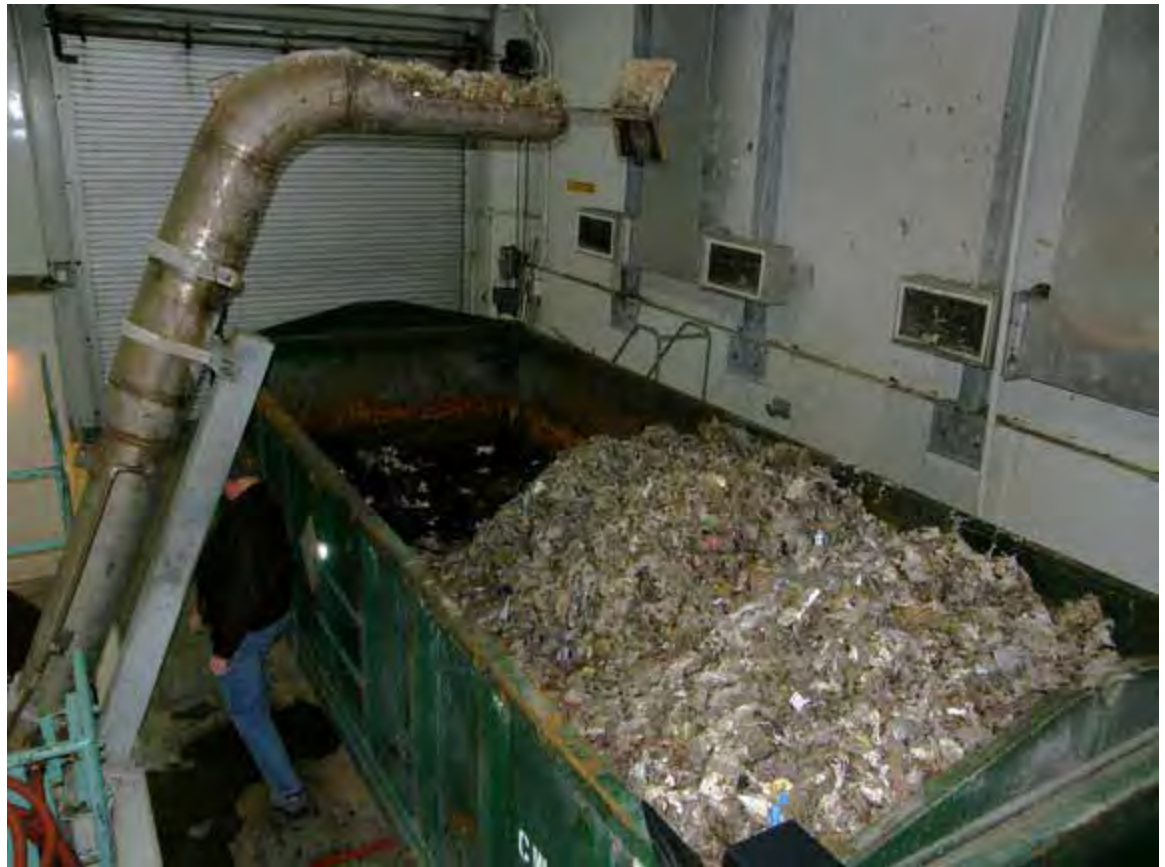
West Point screenings material, which is loosely consolidated, contains fecal material, and is wet
