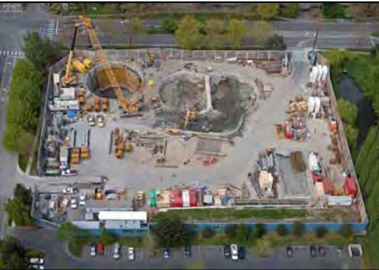
North Creek Portal Construction Site
