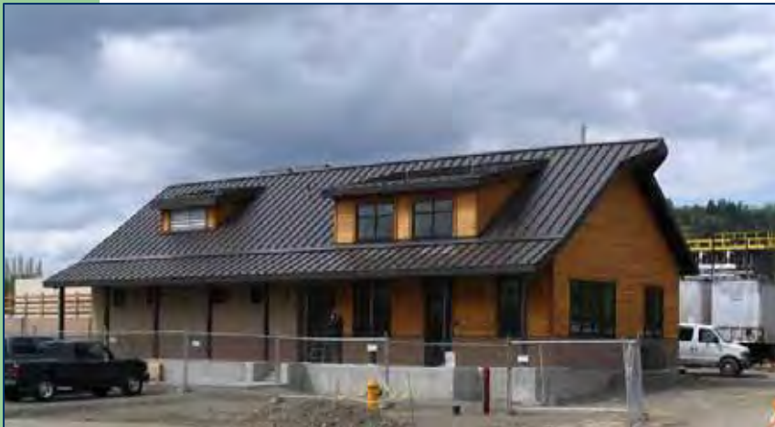
Carnation Wastewater Treatment Plant
