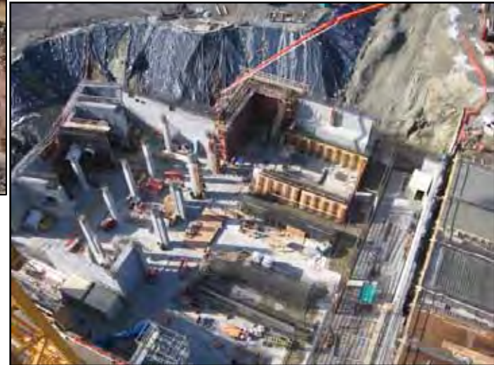
Concrete Work for Brightwater Treatment Plant Headworks Building
